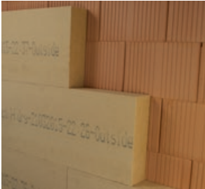
Installation of small-format square edge boards
