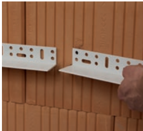
Attach angle rail
