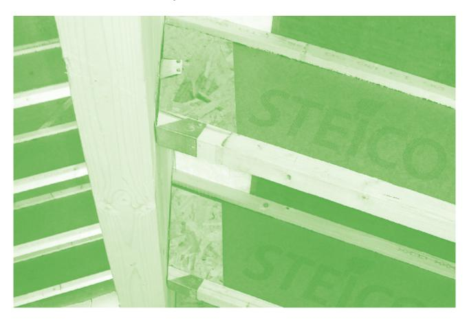
Highly insulated roof constructions are easily achieved with the STEICOjoist. The light-weight joist provides the user a fast and efficient installation for which your carpenter will thank you.
