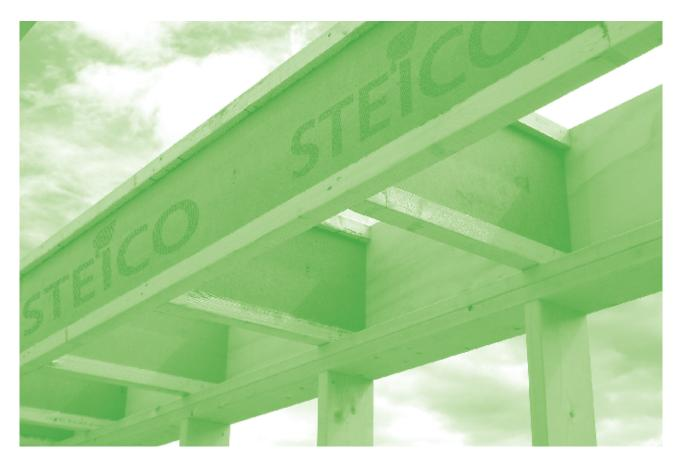
Engineers have long recognised the advantages of an I section in structural elements. Suitable material is only used in those places where it meets the needs, resulting in a slender and economical building element for floors, walls and roofs.
